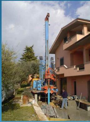
Geothermal bore drilling needs to be carried out by a mast, which is able to face strong bending and torsion strains and has a light and compact design.
